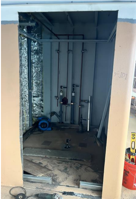
6751 – Restroom Doorway Cut for Door Installation
