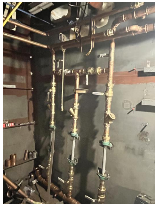
7052 – Manifold for HVAC Tempered Water System
