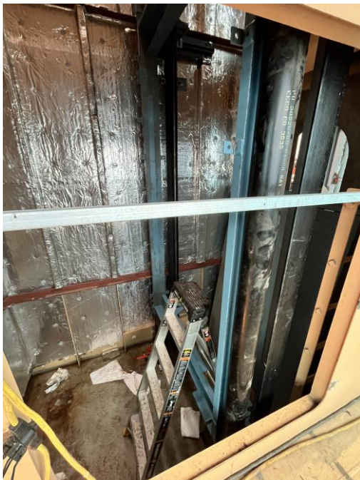
6850 – Installing Elevator Framing Components
