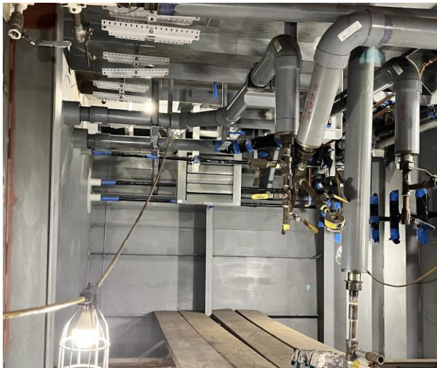
6937 – Piping in Engine Room w/Valves and Painted Out
