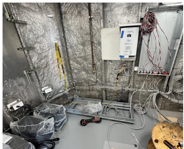
7120 – Setting Panel Box and Back-Up Batteries in Electronics Room
