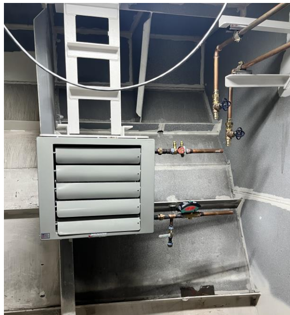
7129 – Unit Heater in a Void Space Being Tied to Tempered Water Piping
