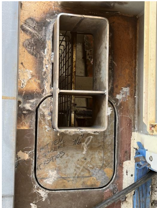
7116 – Installing an Electrical Collar Penetration
