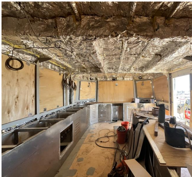
7082 – PH Console In Place After Electrical Chase Work was Completed
