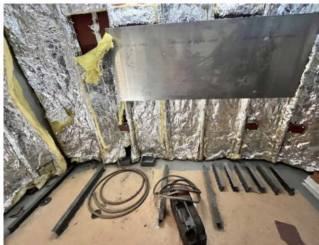
6836 – Foundations & Equipment Backboard in Electronics Room – 02 Deck
