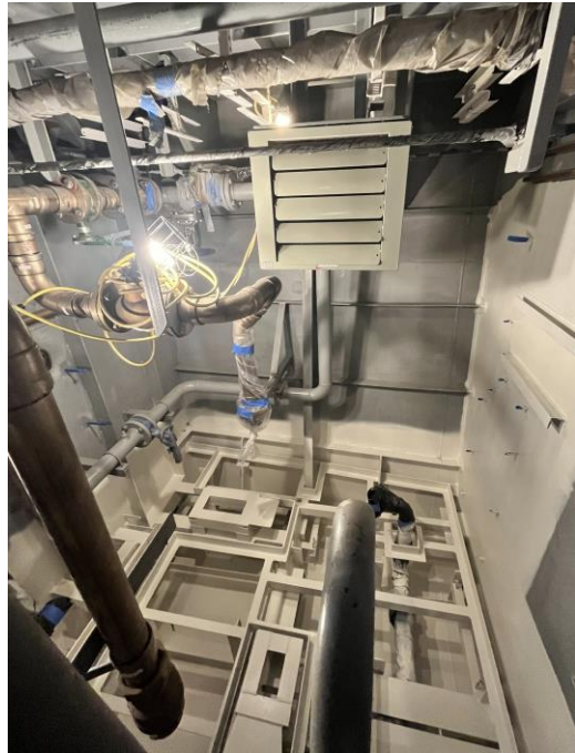
7050 – Unit Heater – Engine Room – Gen Bay
