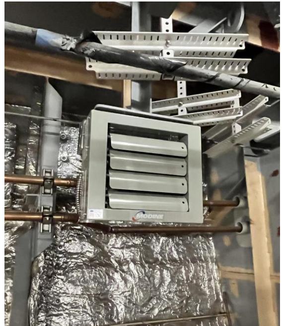
6936 – Typ. Heater in Switch Board Room
