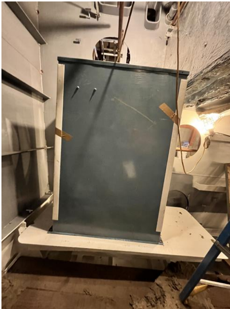
6949 – HPU for Elevator Being Set in Engine Room
