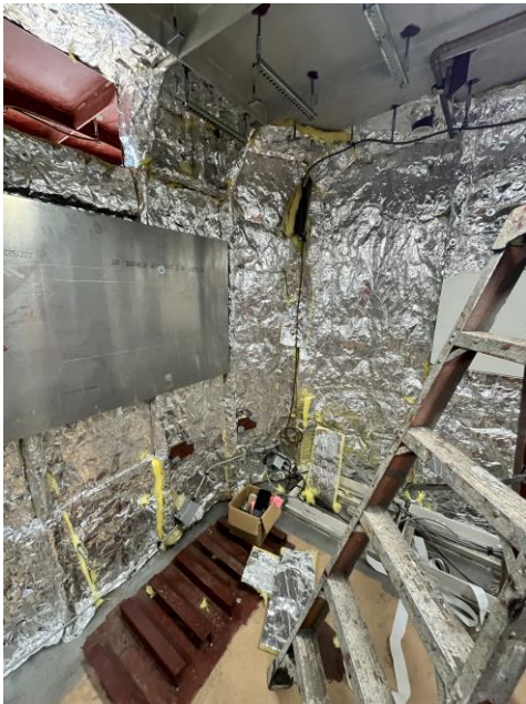
7001 – Insulation in Electronics Room
