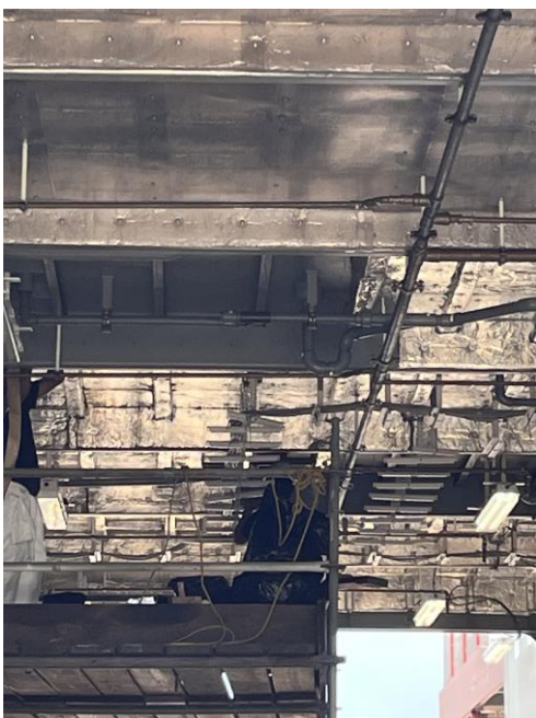
6946 – Lighting & Insulation in Vehicle Alleyway W/Mesh Sheathing in Place
