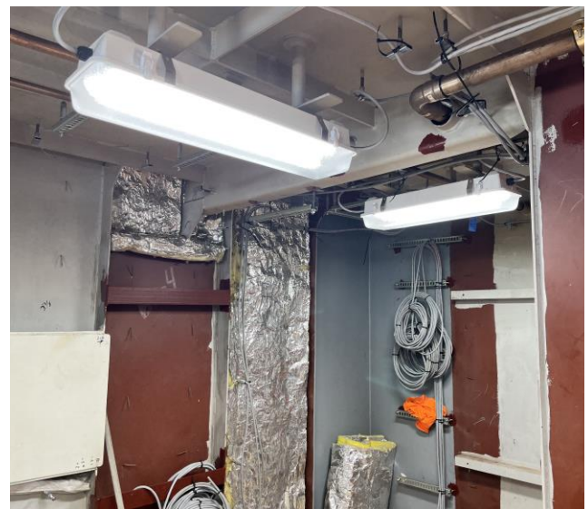
6942 - Electronics Room Wiring & Lights Being Installed
