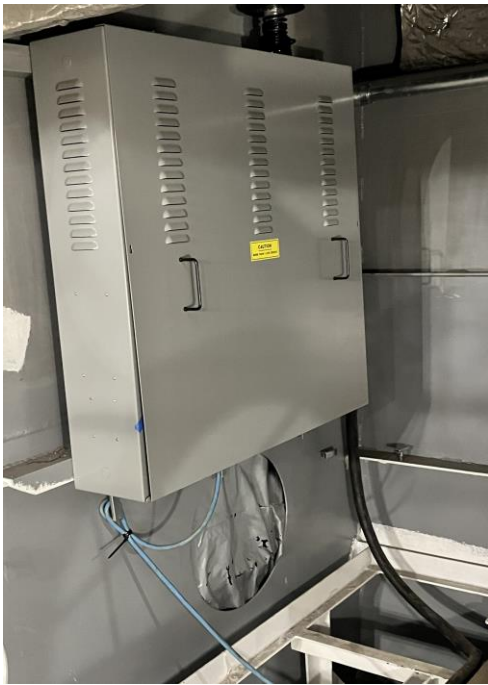
7053 – Control Panel for Elevator
