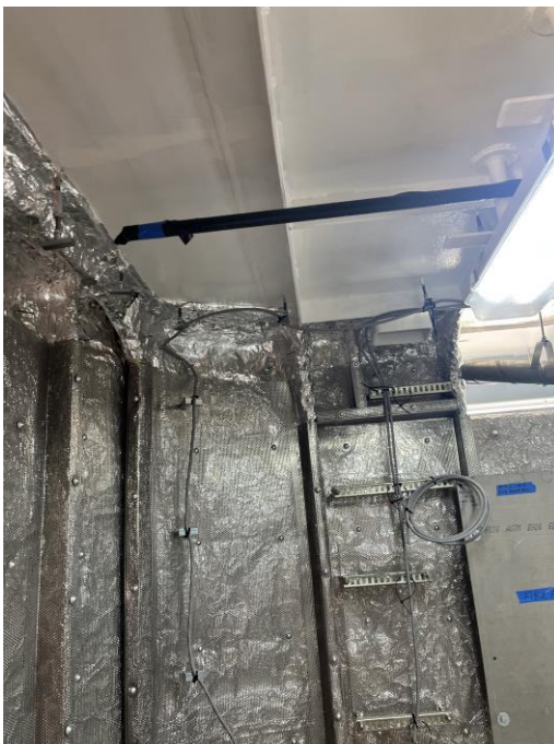
7104 – Insulation w/Mesh Covering in Place
