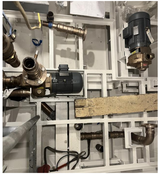
7080 – Fire Main & Bilge Pumps in Engine Room
