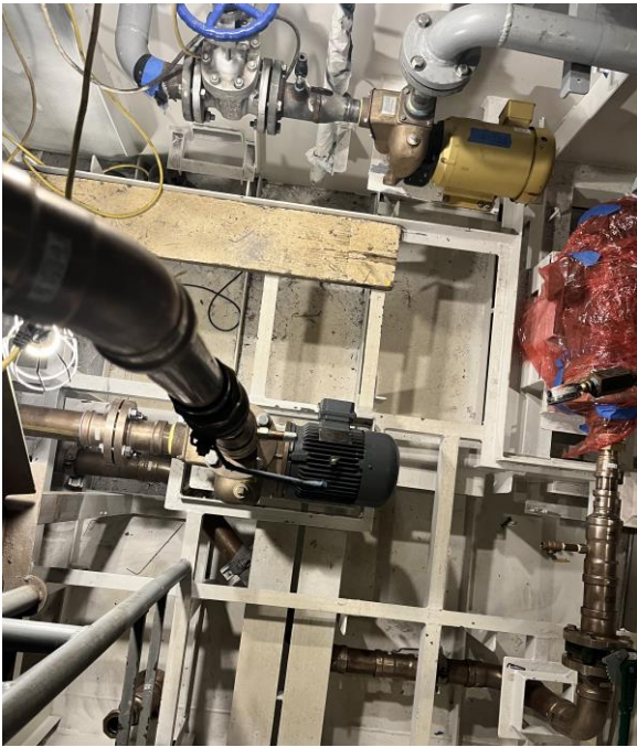
7122 – Bilge & Fire Main w/Sprinkler Pumps
