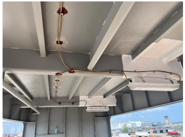
6823 – Typ. Light & Wiring for Covered Passenger Areas
