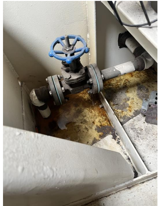
6750 – Bilge Piping Shutoff Valve
