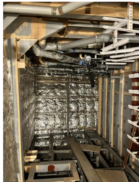
6754 – Piping & Down Comers in Sewer Tank Bay w/Insulation in Place
