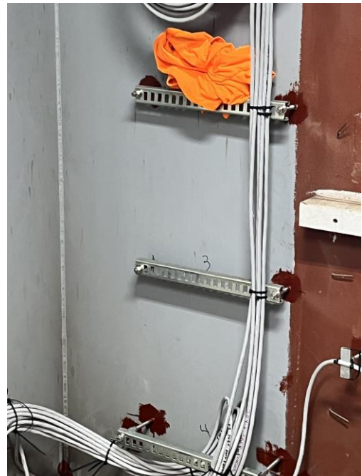
6918 – Installing Wiring in Electronics Room
