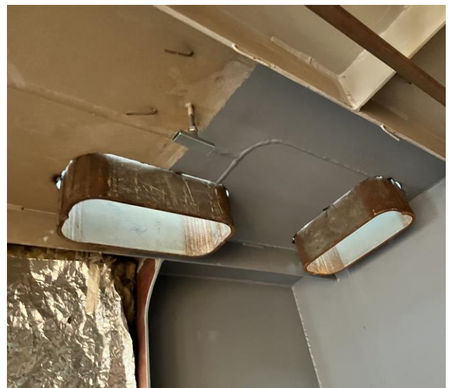
6812 – Electrical Collar Penetration from Electronics Room into Pilot House
