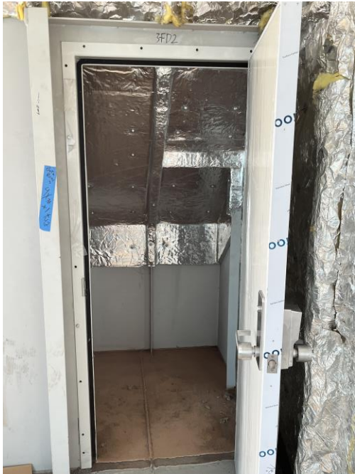
6838 – Door Installed to 01 Deck Crew Locker
