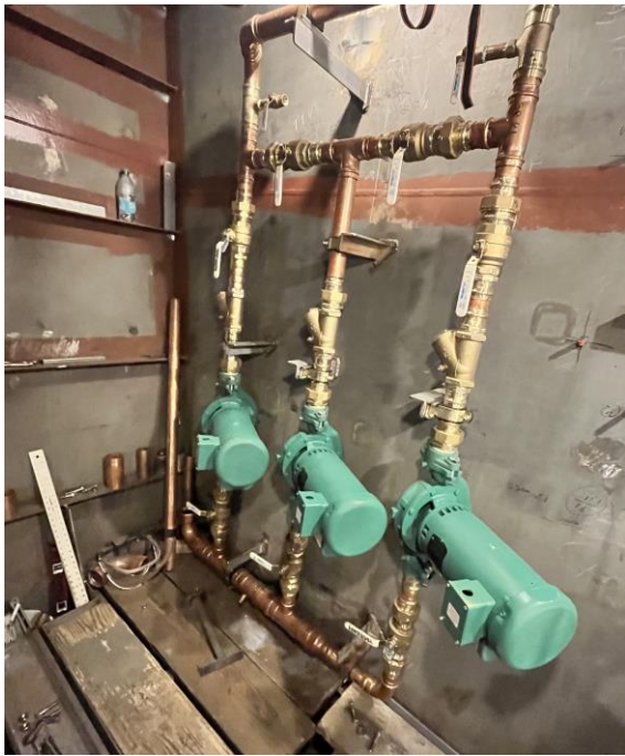
7077 – Circulator Pumps in Boiler Spece
