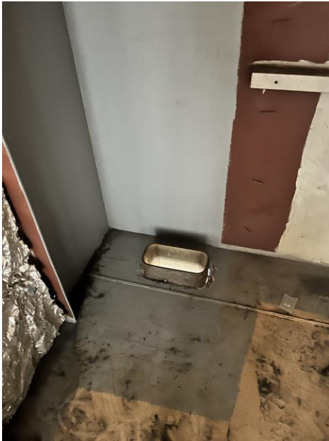
6805 – Electrical Collar Penetration into Electronics Room
