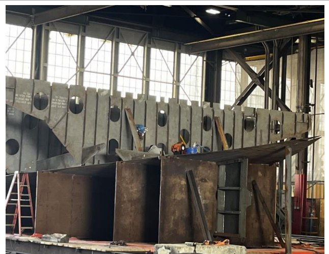
2935 – Module 1 , see point of the bow in bottom plating
