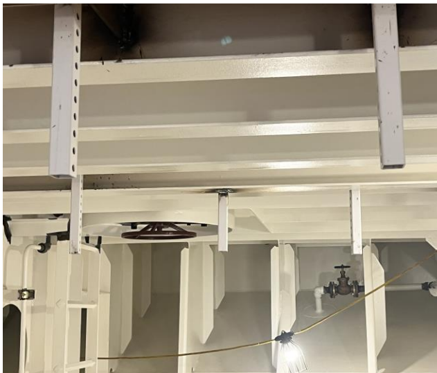
5976 – Access Hatch Handle, Downcomer Lighting Supports and Piping Valves in a Void Space
