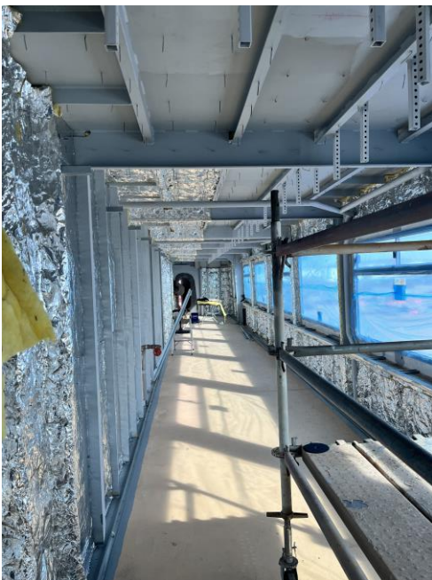
6085 – Port Cabin w/Insulation, Lighting Supports and Insulation Studs
