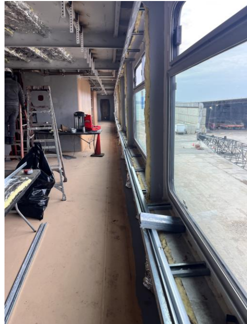
6016 – Starboard Cabin Showing Framing for Window Finishing
