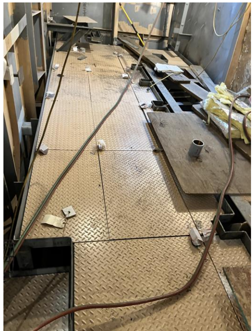
5865 – Installed Floor Plating in a Void Area
