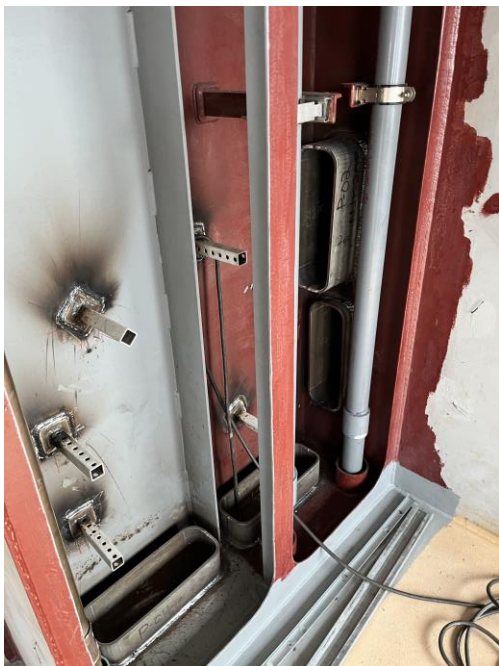
6169 – Electrical Chase with Collars & Supports
