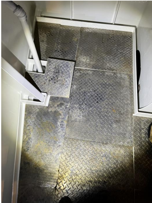
5868 – Installed Floor Plating in a Void Area
