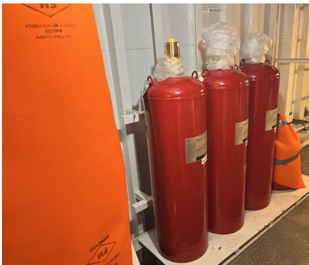
5938 - Fire Suppression System Canisters (Covered to Protect from Other Work Once Installed)
