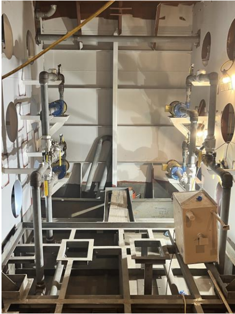
5974 – Machinery Space w/Cooling System Circulation Pumps being Installed
