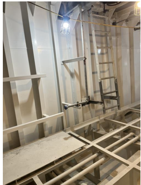
5842 – Typ. Floor Framing in Voids & Engine Room Being Made Ready for Floor Plating
