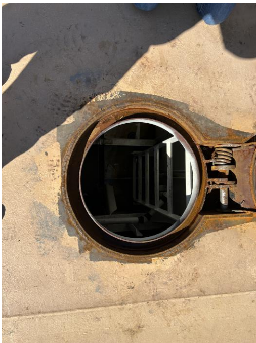
2849 – Hatch Access to a Void Space
