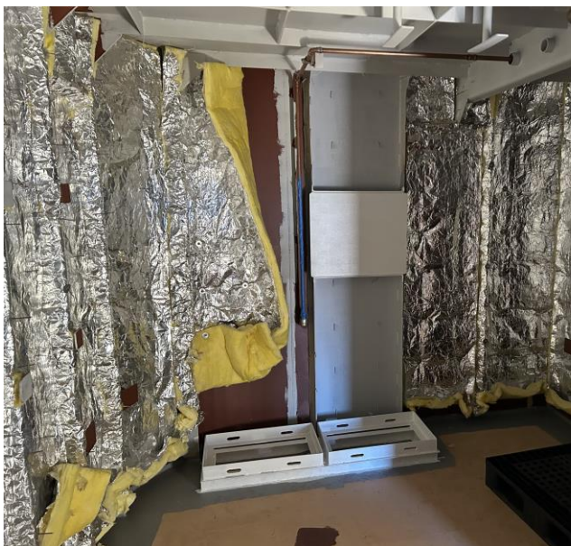
2835 – 02 Deck Electronics Room Insulation
