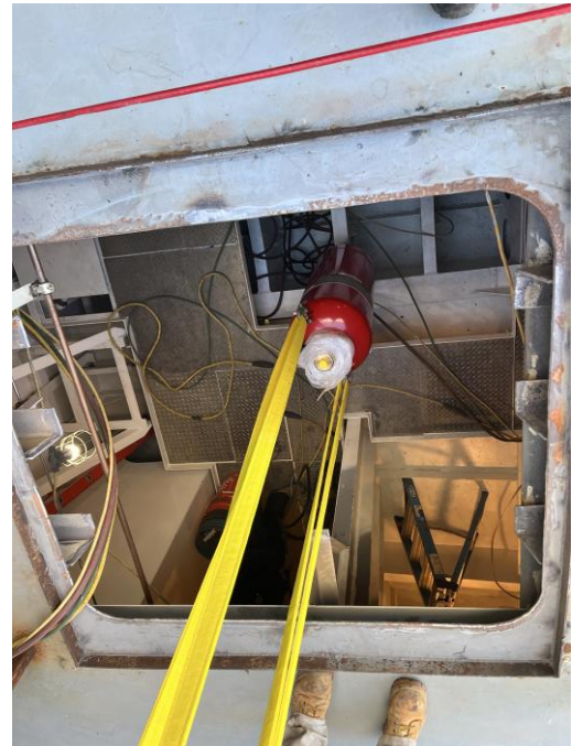
5923 - Installing Fire Suppression System Canister
