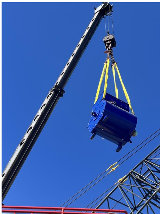
5936 – Lifting Main Propulsion Motor into Vessel
