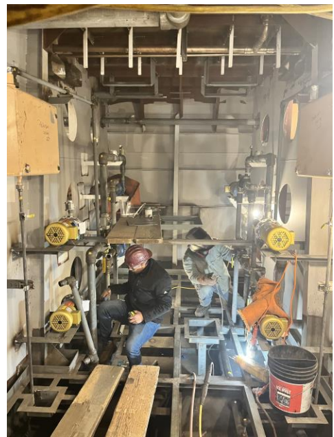
6176 – Machinery Space with Pumps and Piping being Connected
