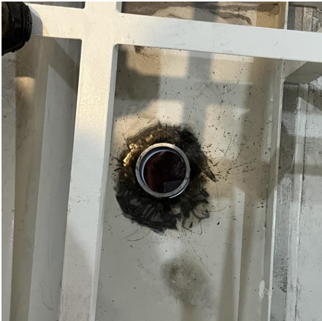
5845 – Bulkhead Penetration from Switchboard Room to Battery Room
