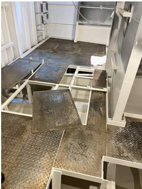
5866 – Installed Floor Plating in a Void Area
