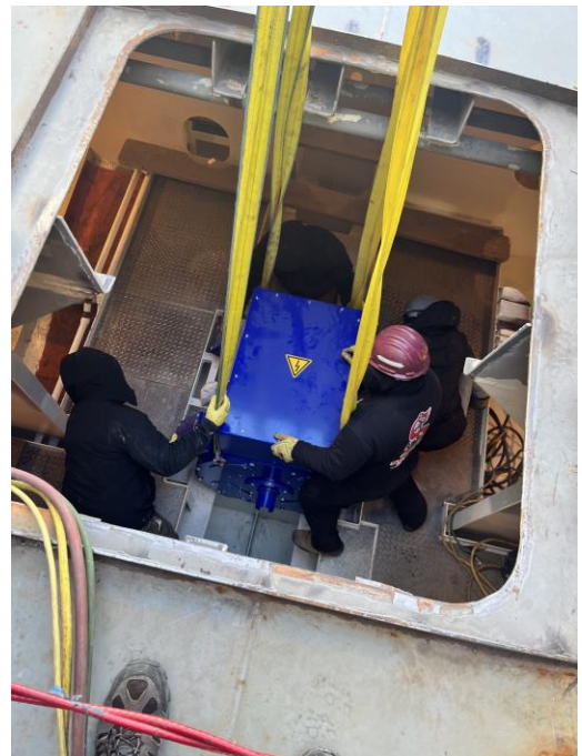
5937 – Lifting Main Propulsion Motor into Vessel
