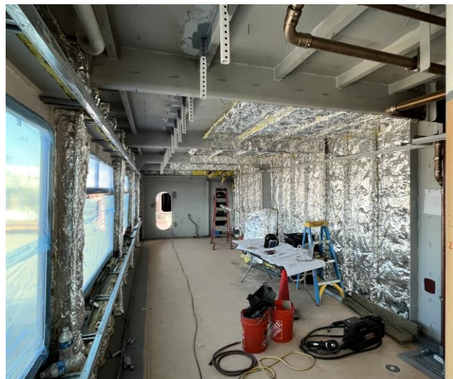
6086 – 01 Starboard Cabin w/Insulation, Lighting Supports, Piping and Insulation Studs
