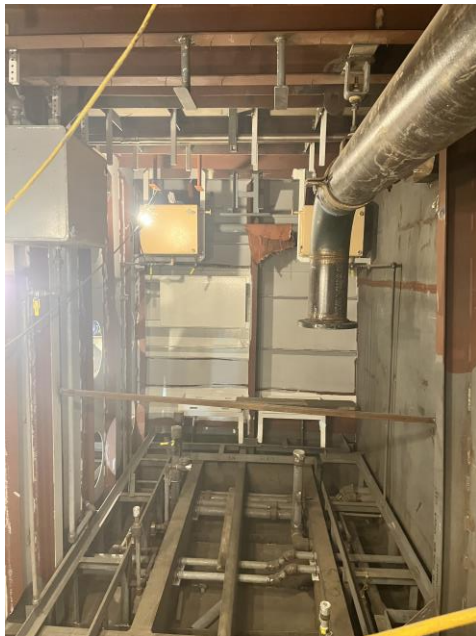
6175 – Generator Space w/Cooling Tanks and Exhaust Piping
