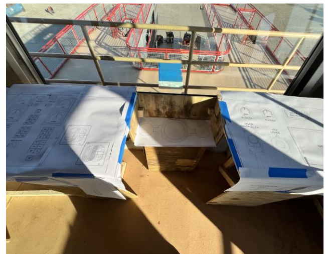
5826 – Pilot House Console Mock-Up w/Location of Controls Laid Out
