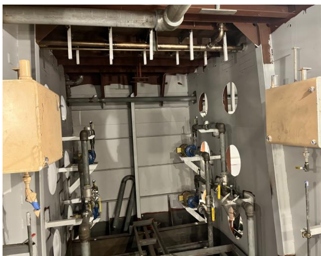
6003 – Cooling Pumps and Tanks in Machinery Space
