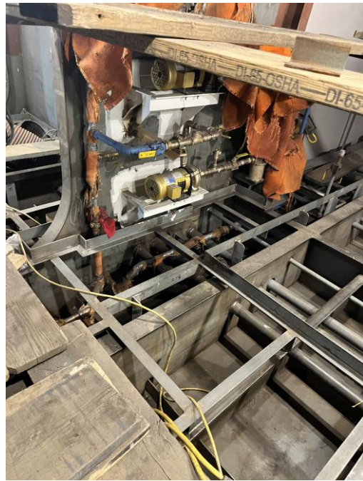
6063 – Circulator Pumps in Machinery Space
