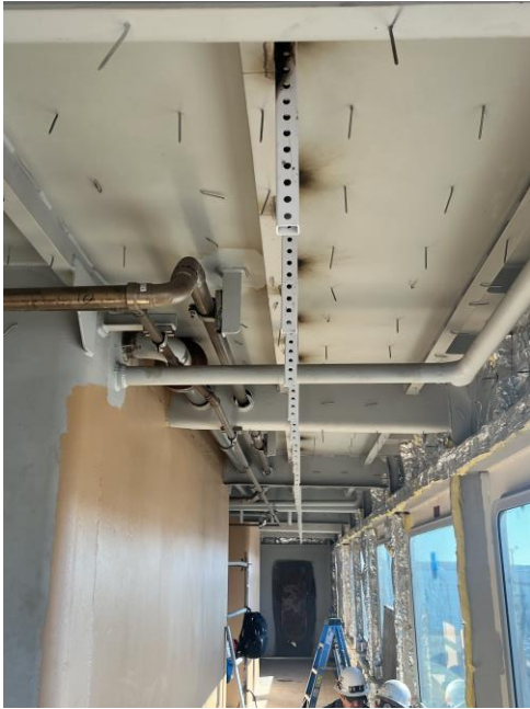
5969 – Starboard Cabin w/ Insulation, Insulation Studs, Piping and Downcomer Lighting Supports
