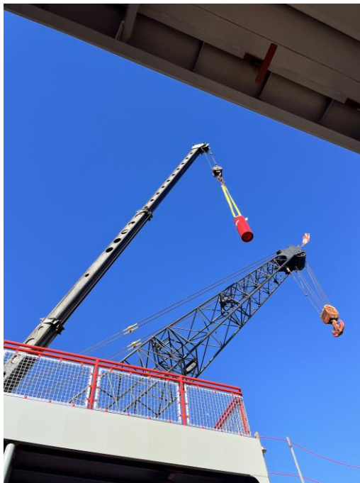
5922 – Installing Fire Suppression System Canister
