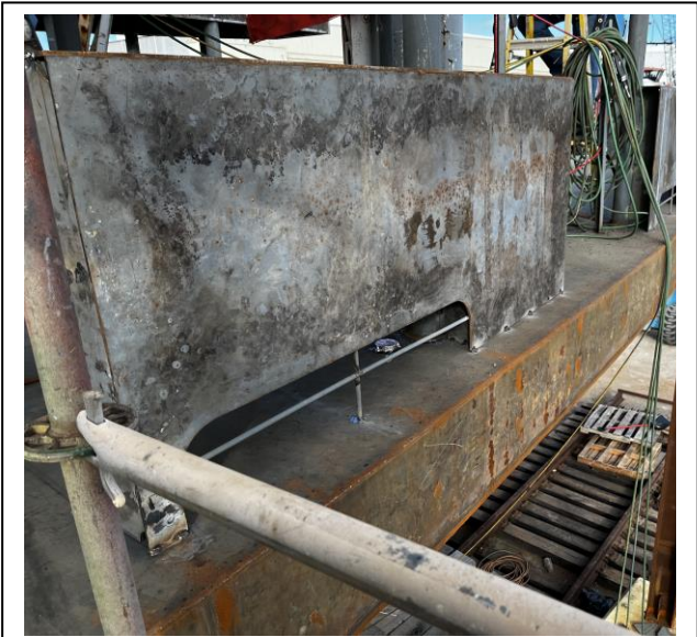
3898 – Bulwark Section on Port Stern End near Anchor Location
