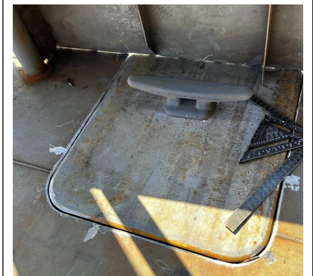
4062 – Kevel Set and Ready for Welding
