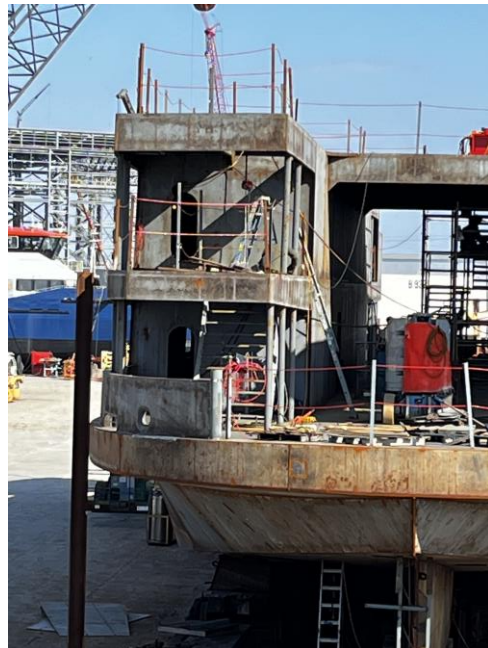
4094 – Starboard Bow End with Stairs from Main to 01 Deck
