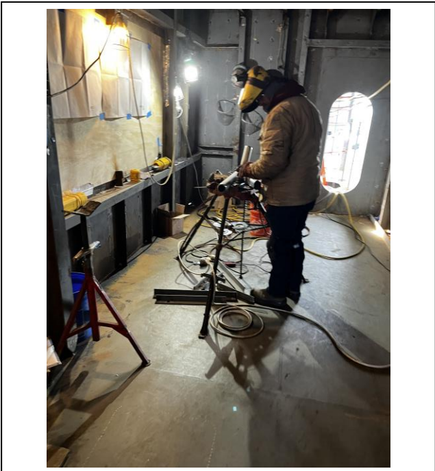
3896 – Fabricating Piping Sections
