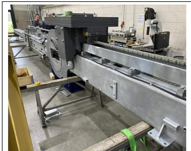
Charger 11 – Constructing Telescoping Arm of Charger
