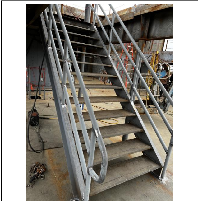
4014 – Bow Starboard Stairs from Main to 01 with Railings
