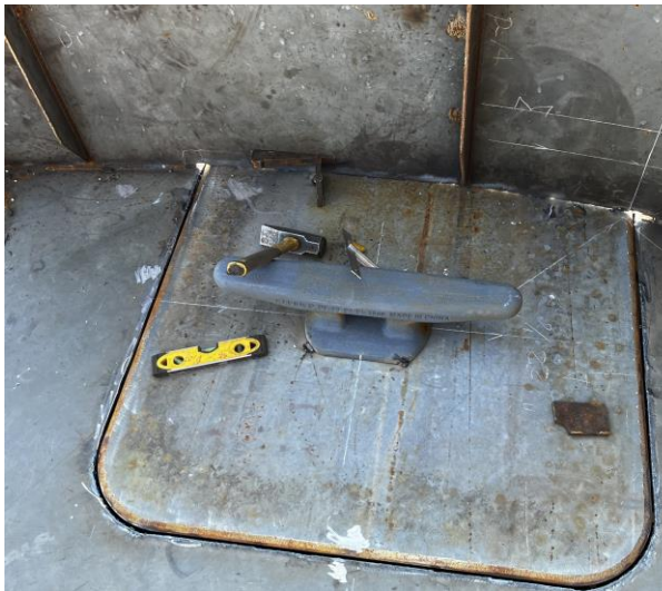
4063 – Kevel (cleat) Tack Welded to Plate
