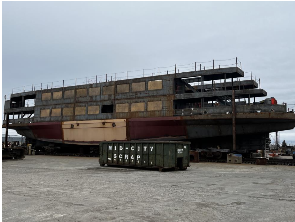
4127 – Starboard Side View of Battery Steele
