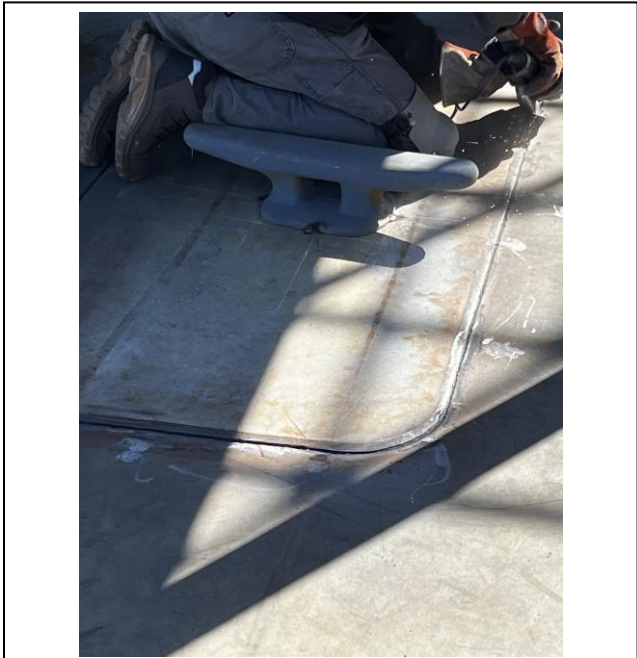
4057 – Kevel Being set and Cleaning Joint for Welding
