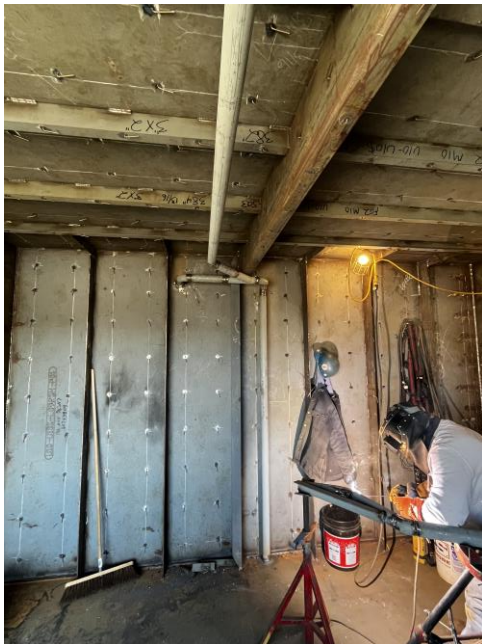
4065 – Piping Fab and Insulation Studs in Engine Room
