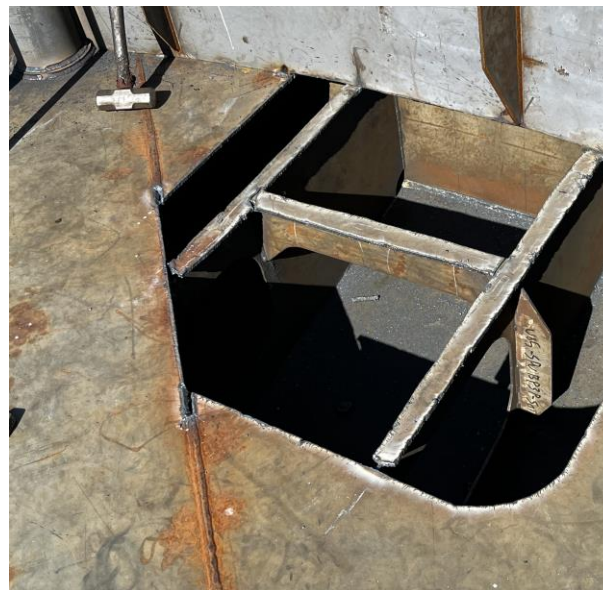
4056 – Opening with stiffeners for Kevel Installation
