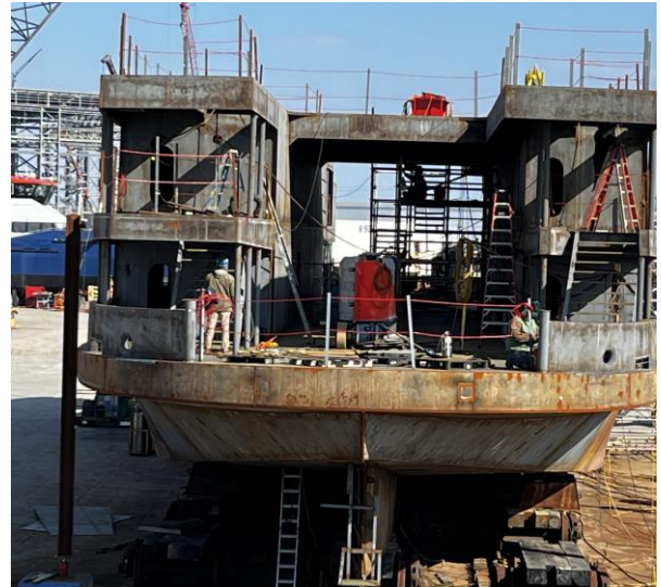
4096 – Bow End with Stairs in Both Sides from Main to 01 Deck
