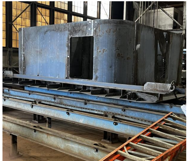
3891 – Deckhouse (Pilot House Base) being constructed upside down
