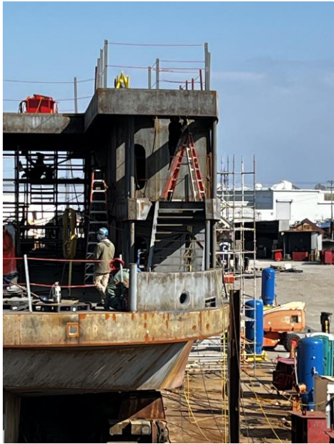
4095 – Port Bow End, Stairs from Main to 01 Deck
