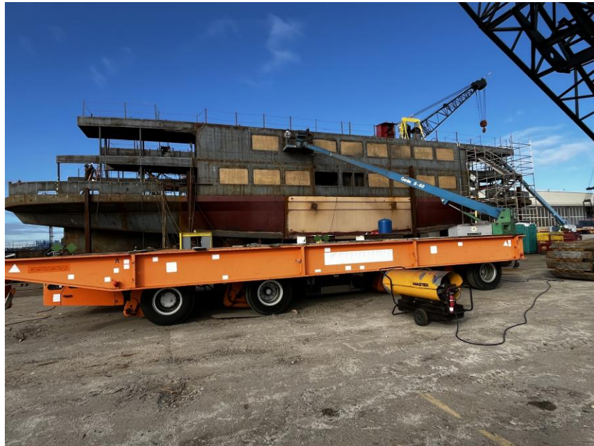
3899 – View of Battery Steel, Starboard Side
