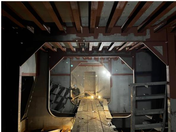
3860 – Inside of Engine Room Space – Note insulation studs welded to ceiling area
