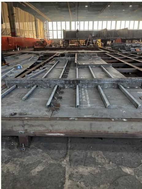
3540 – Deck and framing for modules 6 or 8 which makes up the outside of the 01 deck.
