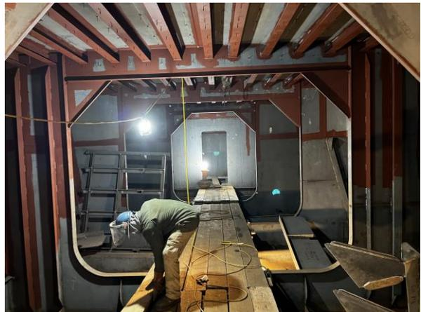
3861 - Inside of Engine Room Space - Note insulation studs welded to ceiling area
