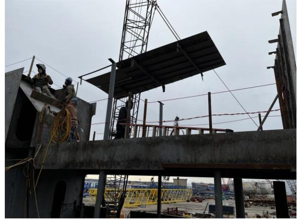
3828 – Setting Module 9 deck plating (02 Deck) on stern of vessel
