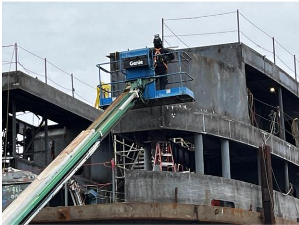
3841 – Working on Charger Socket Enclosure on 01 deck starboard stern.
