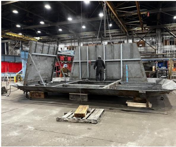
3831 – Placing Pilot House Bulkheads – house is being constructed upside down.
