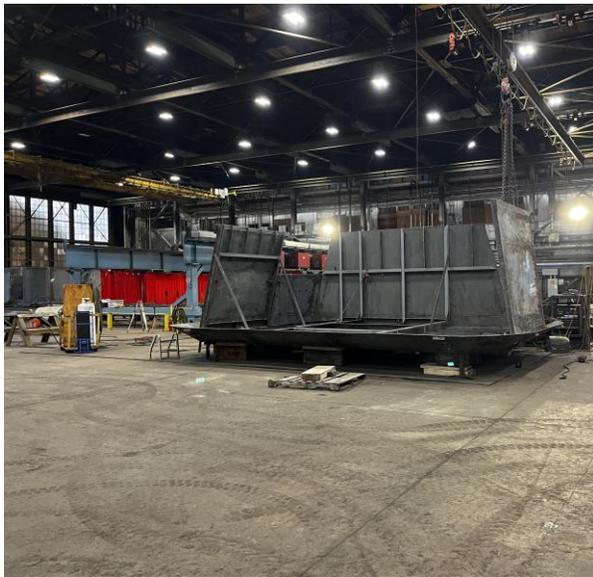
3833 - Placing Pilot House Bulkheads – house is being constructed upside down.
