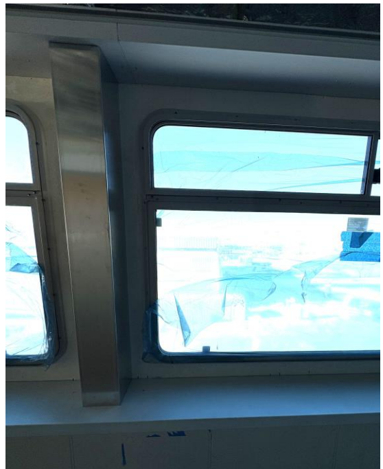
9339 – Doing Finish Work Around Cabin Windows
