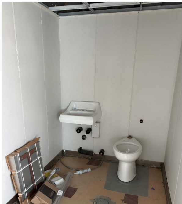
9270 – Restroom Fixtures Being Installed
