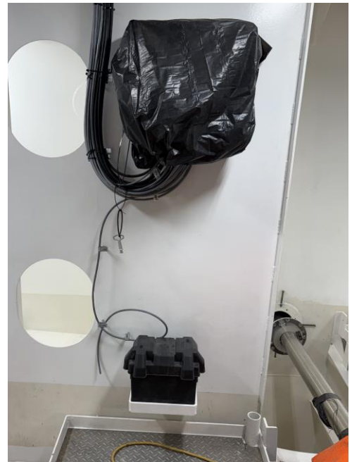
9585 – Battery for Ultra Fog Water Mist System (Control are Covered w/Bag)
