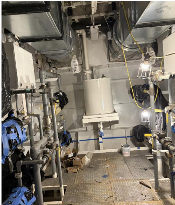
9251 – Lube Oil Tank in Pump Space of Engine Room
