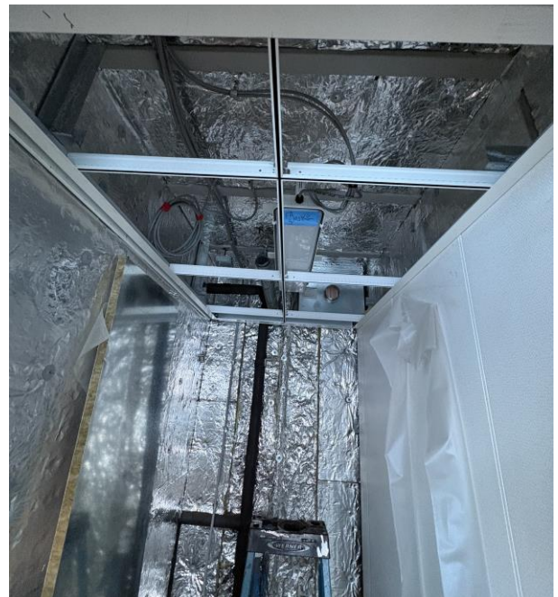
9133 – Ceiling Grid being Installed in Cleaning Locker
