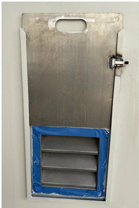
9286 – Vent w/Cover Prepared for Painting
