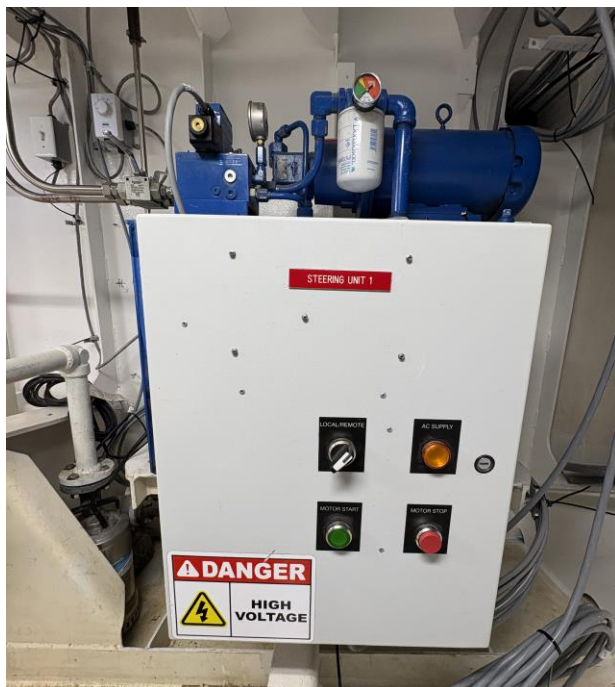
9508 – Typ. Steering Unit Control Panel
