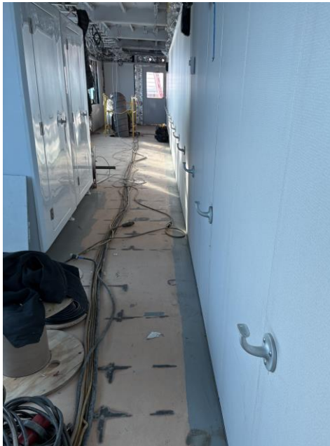
9301 – Handrail Support Being Installed in Main Deck Port Cabin
