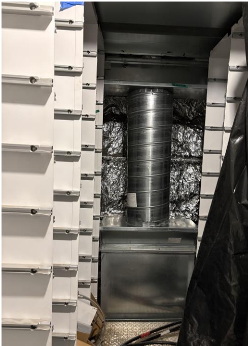
9335 – Ventilation Ducts in Battery Room
