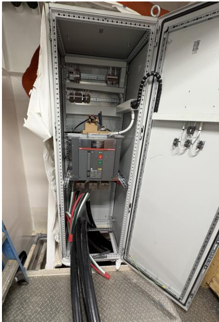
9088 – UPS Cabinet, Installing Wiring
