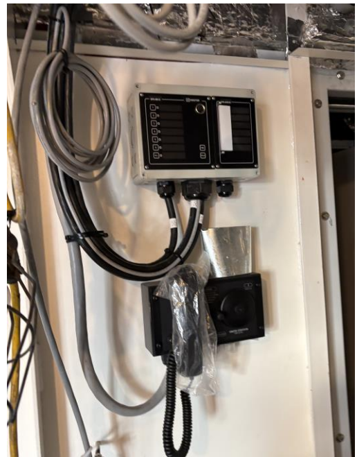
9347– Typ. Communication Station throughout Vessel
