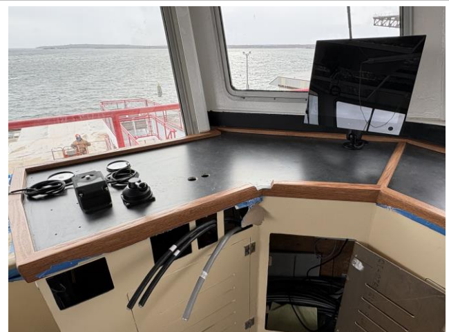
9313 – Bow PH Console w/Steering Controls Being Installed
