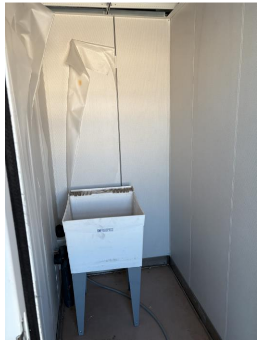
9300 – Utility Sink Being Installed in Cleaning Locker
