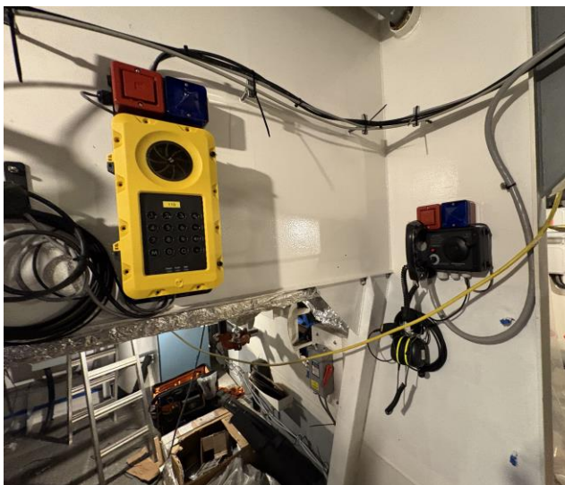
9135 – Communication Systems in Engine Room
