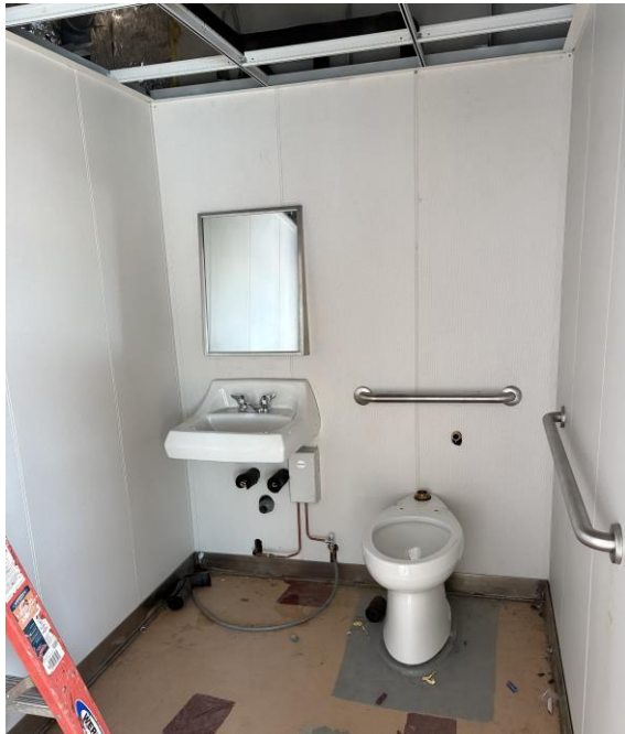
9273 – Restroom Fixtures Being Installed
