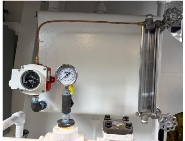
9495 – Expansion Tank w/Gauges & Site Glass
